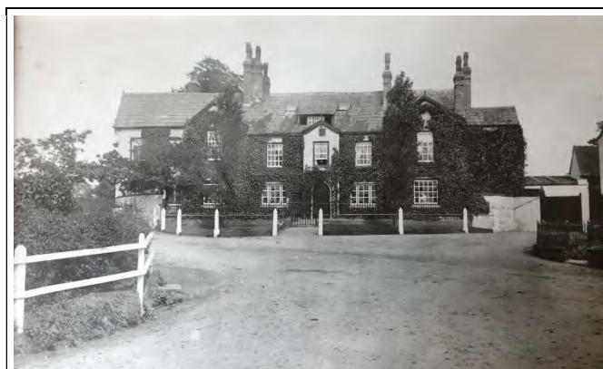
Former Boundary Treatment of Ollerton Hall
