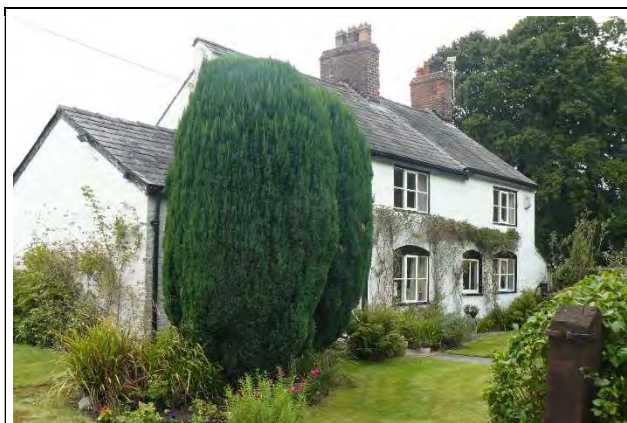
Ollerton School House
