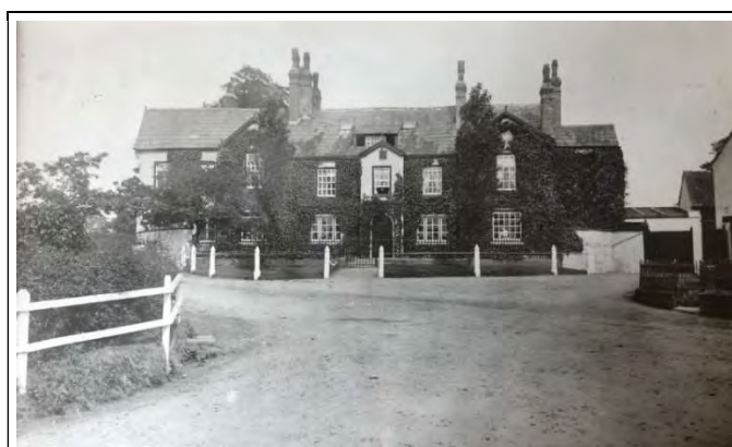
Ollerton Hall Front Elevation ca. 1914
