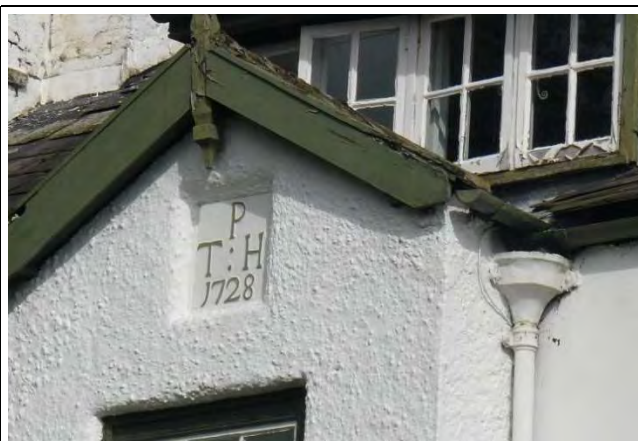
Original Casement Windows, Ollerton Hall
