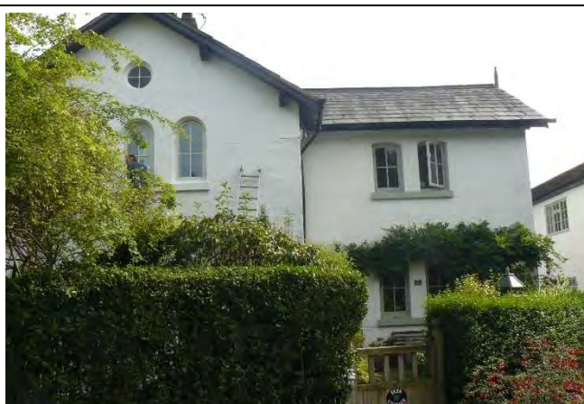
New Windows in Original Openings
